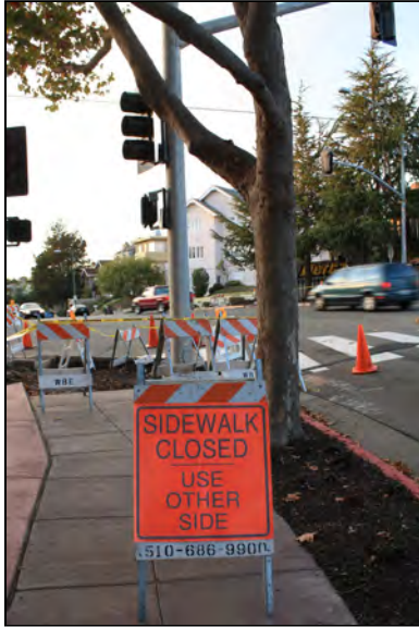
New signal installation, Rose and Grand
